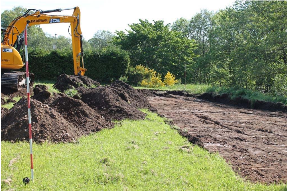
Figure 6: LK15 trench during machine stripping
