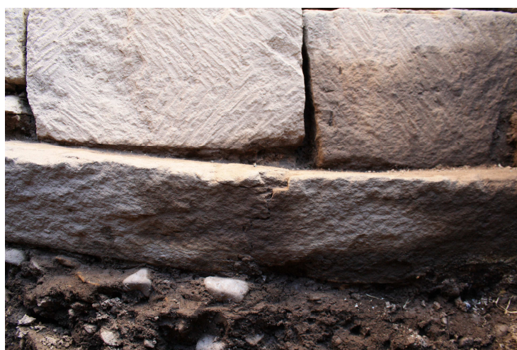
Fig 5 Detail of toolmarks on tower plinth 4707 (above), and lack of them on early structure 4711 (below)
