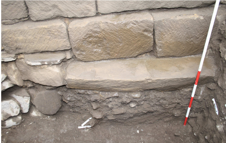
Fig 7 The early structure 4711, showing different foundation from boulders of 4723, and jumbled stonework of intersection with plinth of tower. Note early Burial 4 (white tags) running under foundations.
