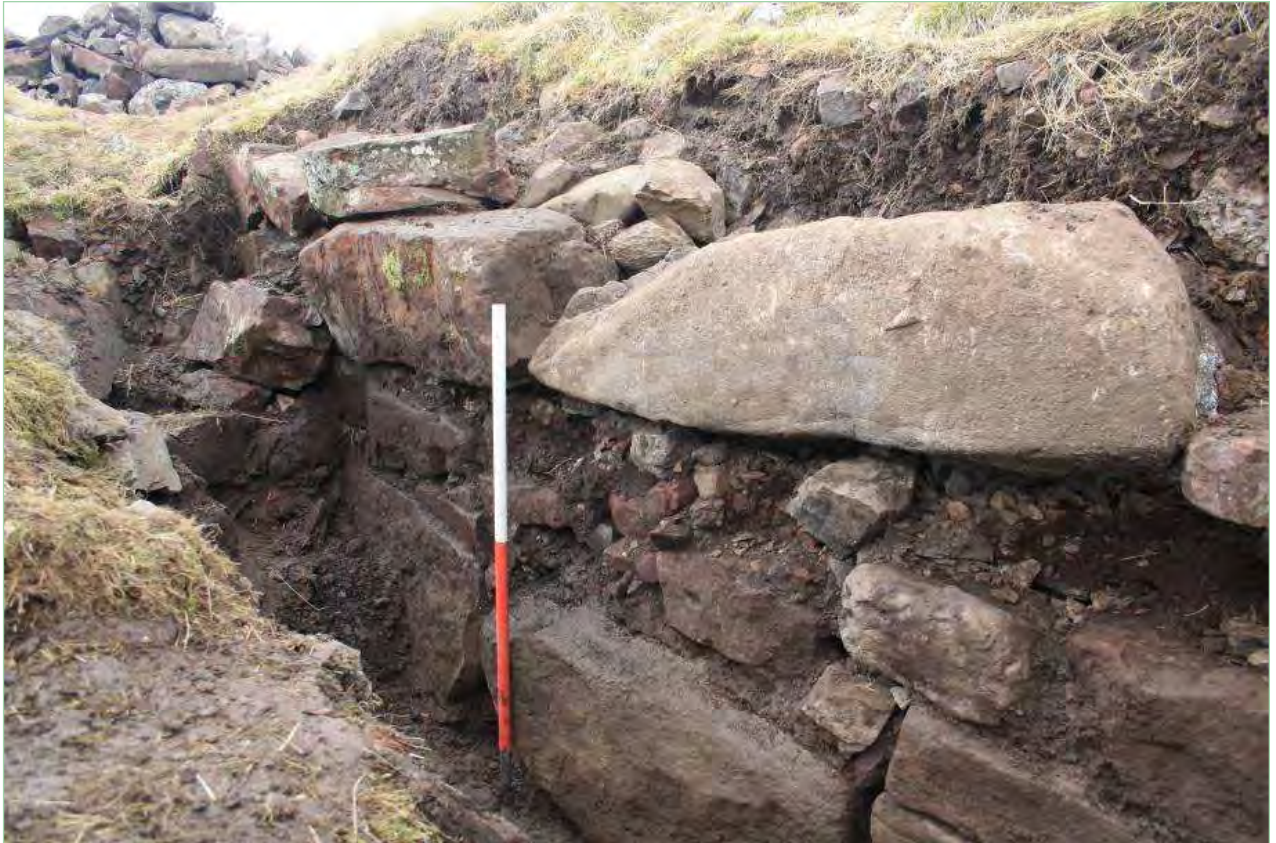
Plate 27: Outer wall face of the inner enclosure, from the NE
