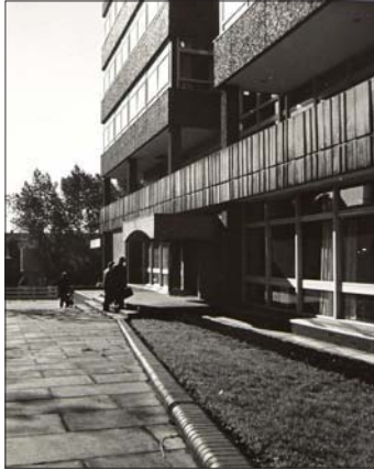
The Adam Smith Building was built in the 1960s. The Department moved into it in 1968. Source: Glasgow University Archives, PHU/6/3.
