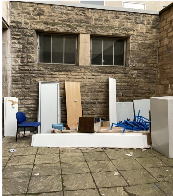
Combustible material stored next to building.
