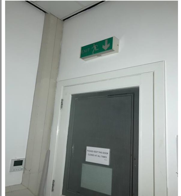
Example of older type emergency lighting.
