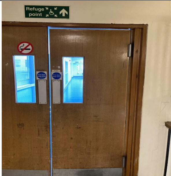
Evidence of fire door requiring maintenance and non-compliant hinges.
